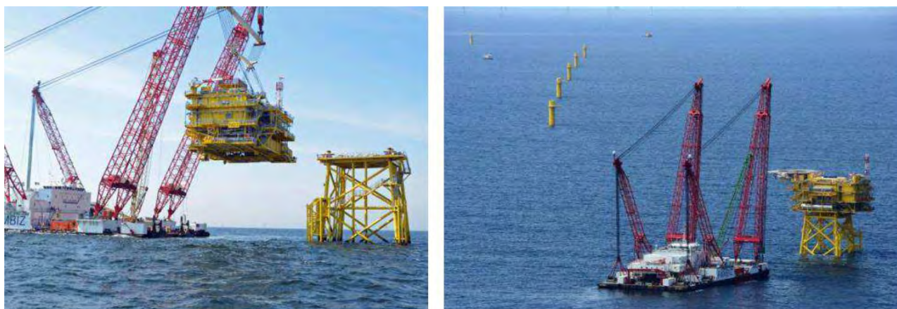
Figure 60 Installation of topside
