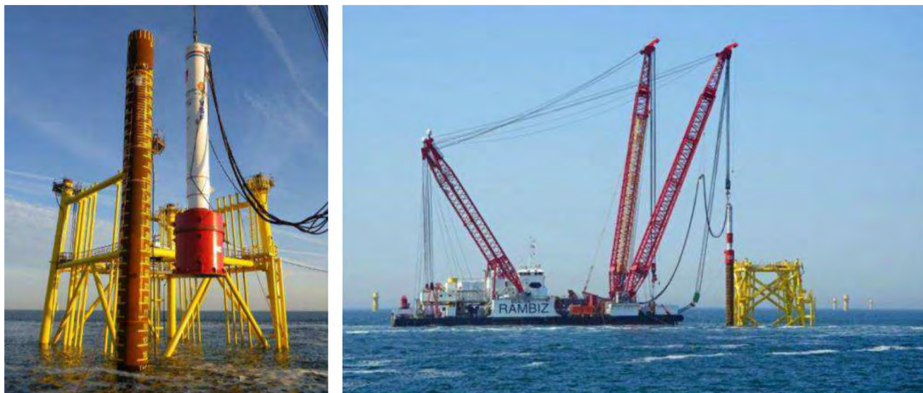
Figure 59 Piling of jacket
