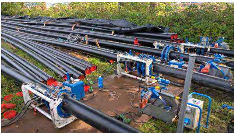
Figure 27 Welding of HDPE ducts
