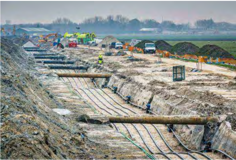
Figure 14 Example of a trench using the preferred trench configuration method
