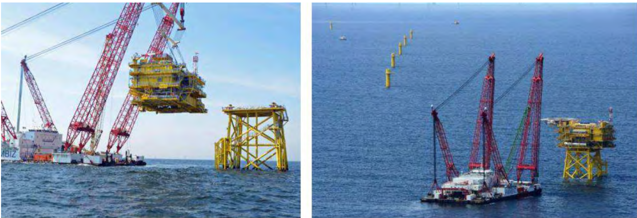
Figure 60 Installation of topside
