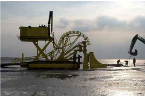
Figure 51 Vibration plough on tracks
