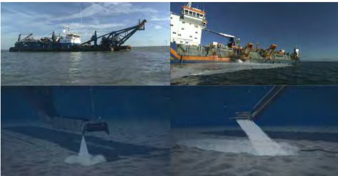
Figure 44 Mass flow excavation by a converted Suction Dredger or Hopper Dredger
