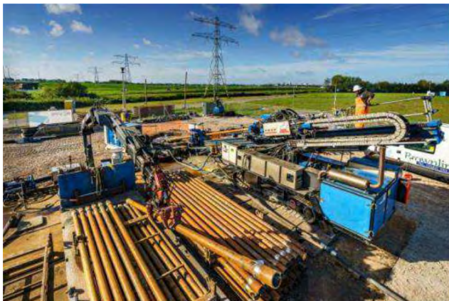
Figure 26 Example of HDD entry and exit point
