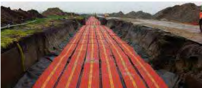
Figure 18 Open cable trench, after the pull-in of the cables
