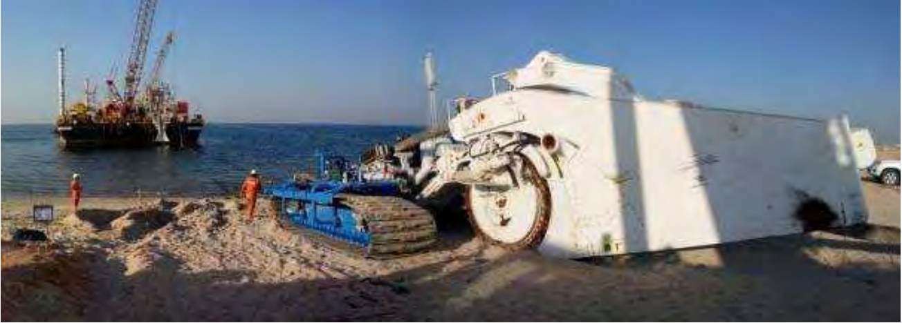
Figure 41 TM04 Wheel cutter cable trencher
