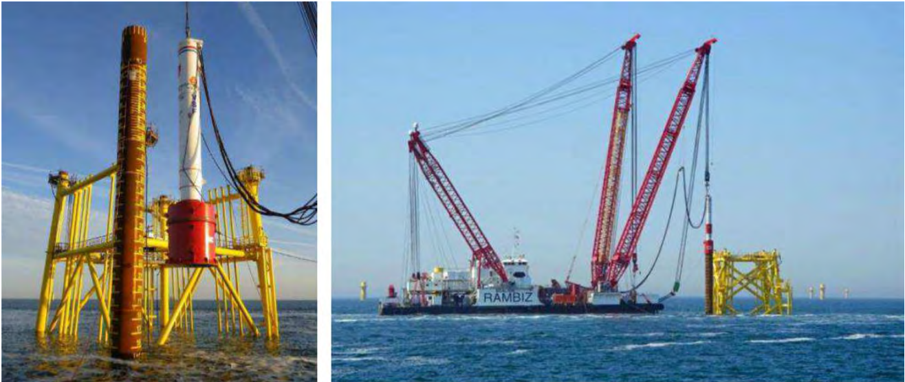
Figure 59 Piling of jacket
