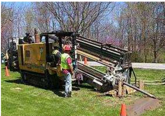
Figure 29 Example HDD rigs - [left] midi rig - [right] maxi rig
