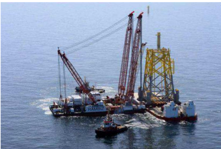
Figure 58 Installation of jacket
