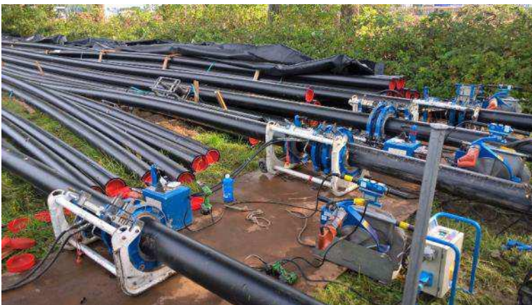
Figure 27 Welding of HDPE ducts
