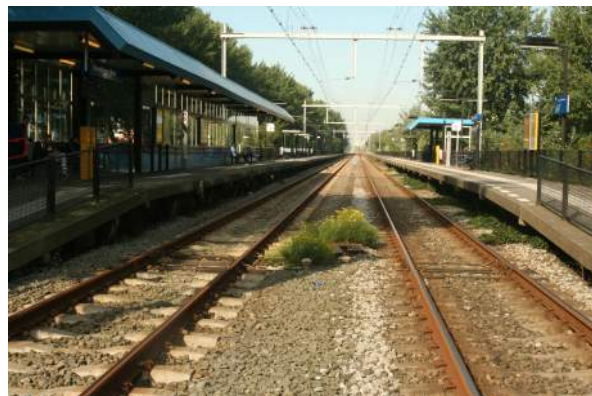
Figuur 4.14 Station Vlaardingen West.
